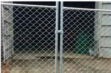
⊕ Fence panel assembled with tension bars
